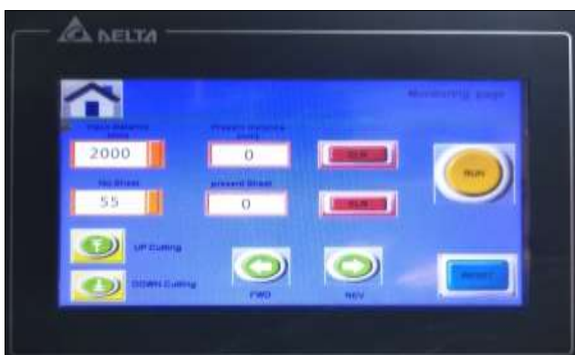
Fig 11: Control desk panel
